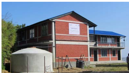
One of the two tanks in Shivalay School, this tank is finished and collecting water.
