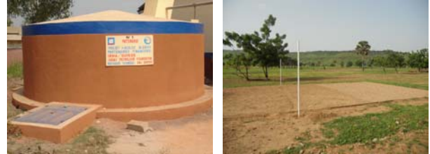
One of the 14 water tanks built and Bogou School's new volleyball court.
