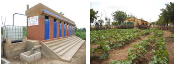
One of the new toilet blocks in Agbodji School and the vegetable garden in Dampiong School.
