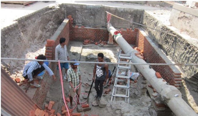
Figure 1 Construction of a 50m 3 underground tank ©IRHA-GUTHI
