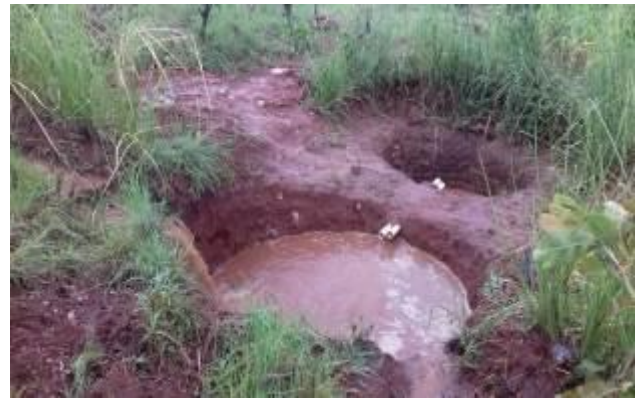
In general it is recommended to make round pit which are stronger. Make the sides a bit sloped so there is less danger of collapsing.
