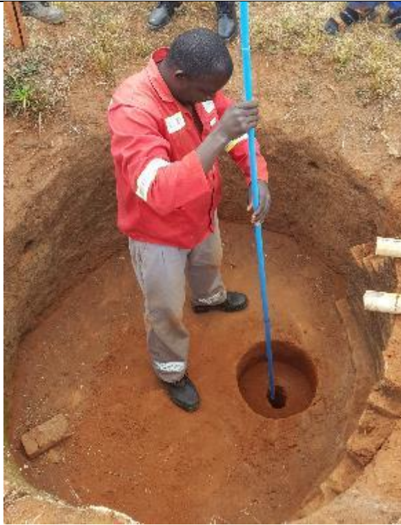
Installing the PVC pipe
