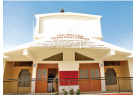
Front view of a Sulabh Toilet Complex at Kabul.
